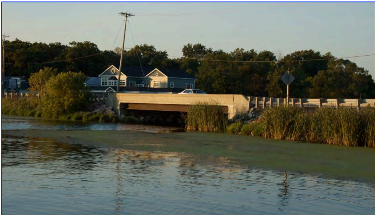
Delavan Lake at Highway 50
