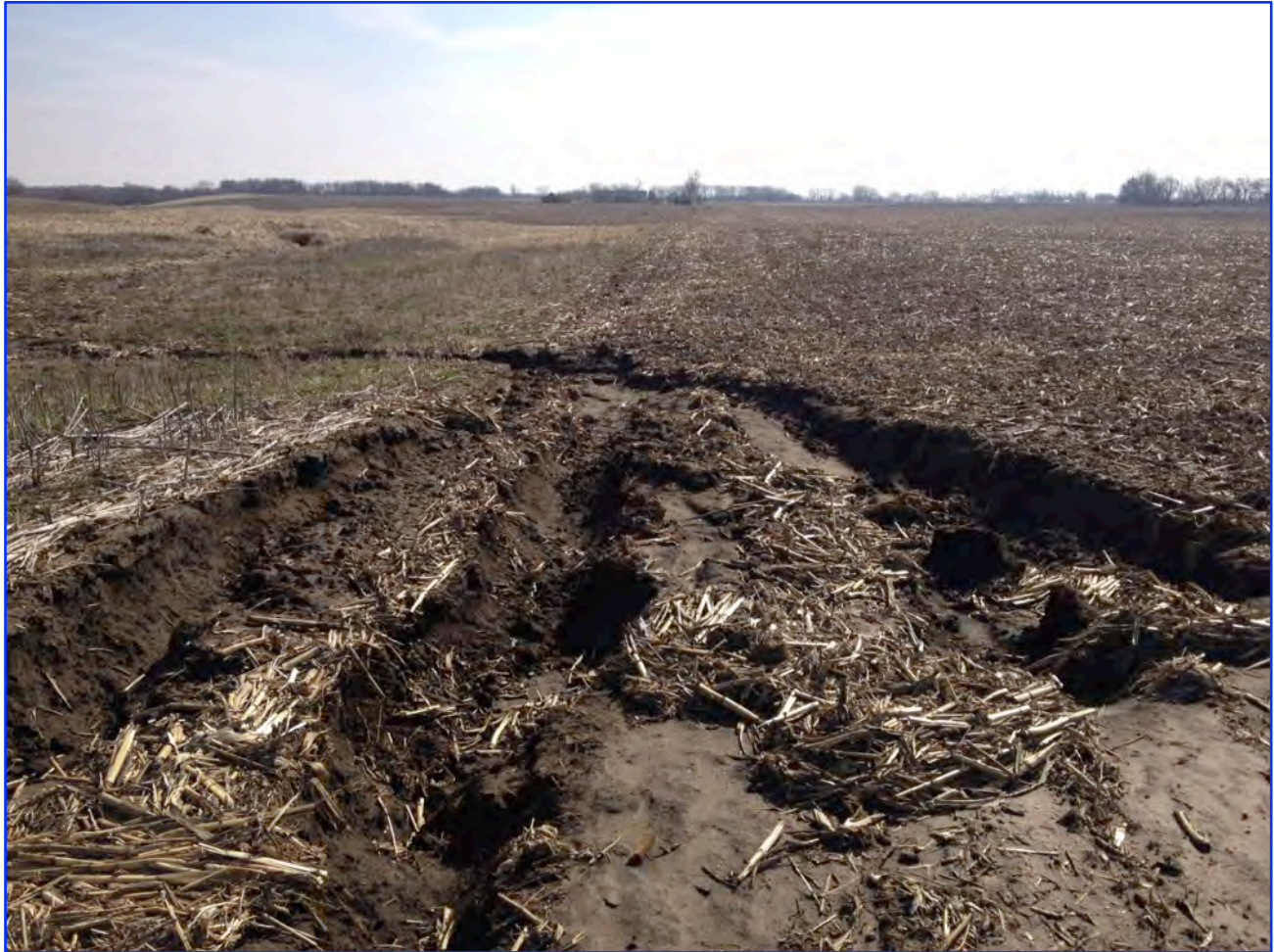
Figure 17 – Examples of Eroding Gullies
