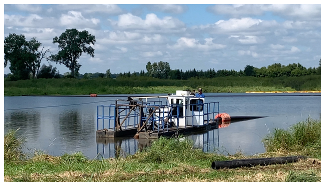
The dredger on it's first pass on the east pond
